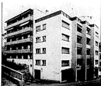
Avenue Recordon 16 Lausanne
