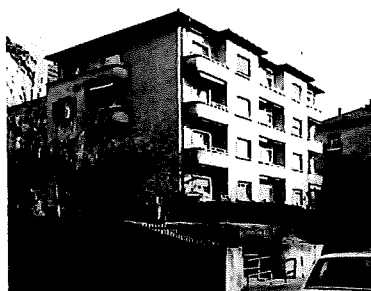
Avenue Sévery 14 Lausanne
