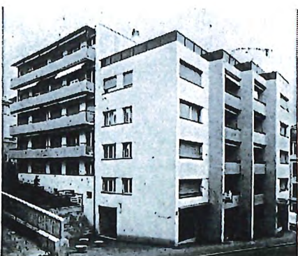
Avenue Recordon 16 Lausanne
